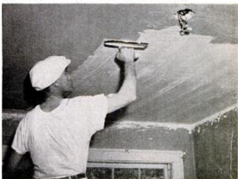
Finish coat can be applied 24 hrs. after base coat. Photo above shows start of finish-coat application, beginning at side of room and working toward center
